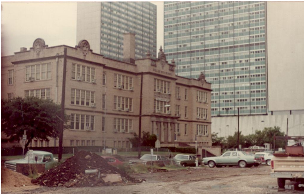
Images of the site. The site in the 1980's (bottom)
